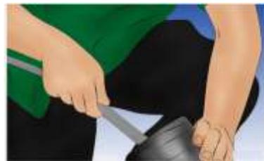
**Clean the vent line regularly** – it is very important that the vent line (from the wall behind the dryer to the outside flap) is not restricted or clogged up with lint. This increases chance of a dryer fire.
