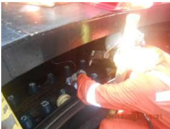
Turret working location
