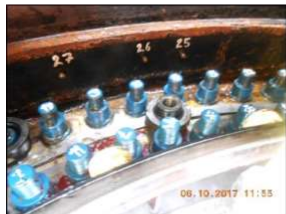
Tensioner part trapped between bearing race stud bolts
