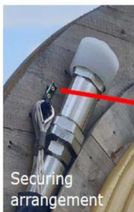
Picture 1 shows how 2nd end termination head end was secured
