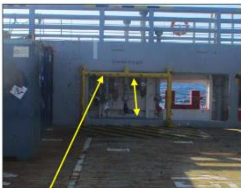
Basket swung under protective rail
