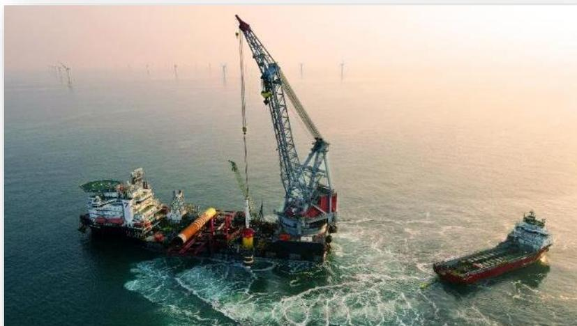
Figure 12 – Pile installation on DP
