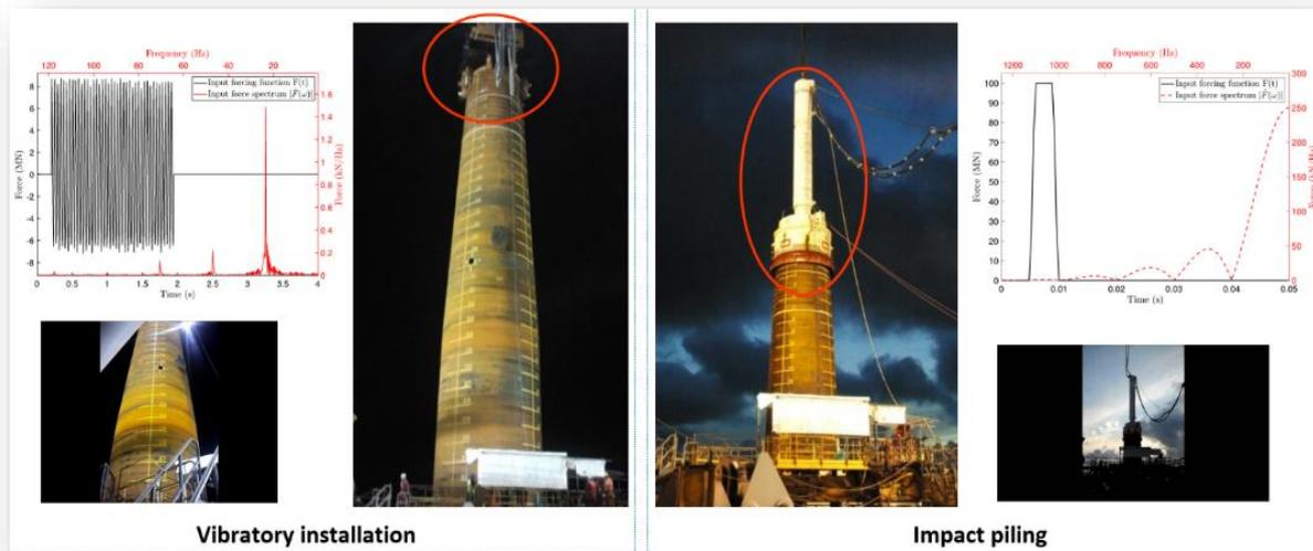
Figure 53 – Noise from vibratory and impact piling
