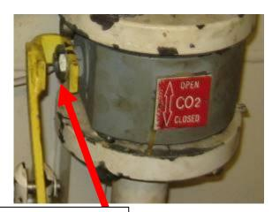
Spindle remained in the closed position whilst the handle was in the open
