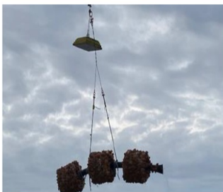
Riser section recovery
