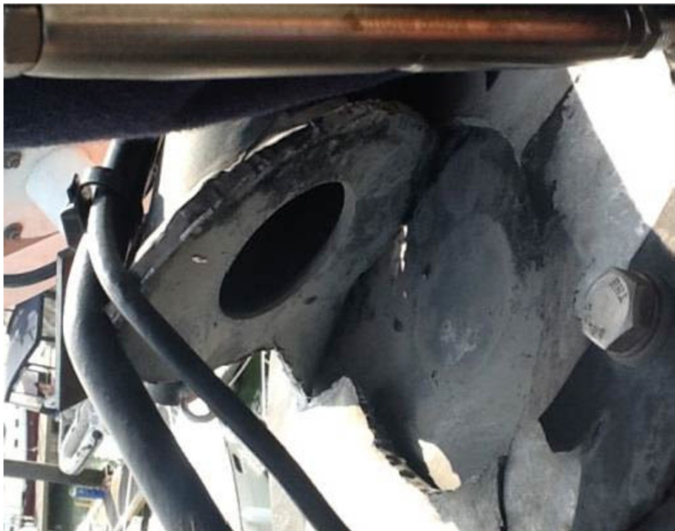
Mast damage following the first incident
