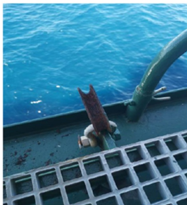
Lack of clearance (cordage – deck strong point)
