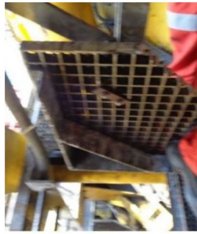
(Right) Intact manhole door raised, showing bracket in upright position. The dropped object bracket was in similar position due to previous unreported incident.
