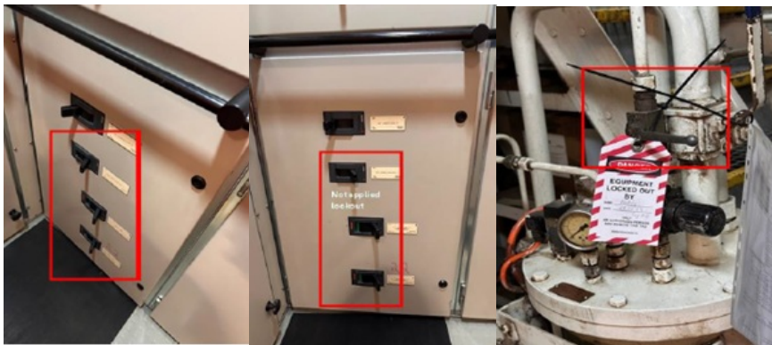
Case 2: No mechanical valve lock out was applied on the equipment
