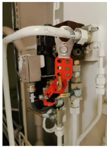
Picture of bridge IAS control left and properly isolated control valve hydraulic flow right
