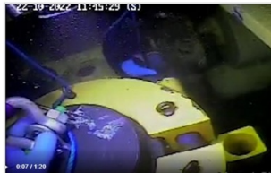
Image 2 – Diver loosening bolts
