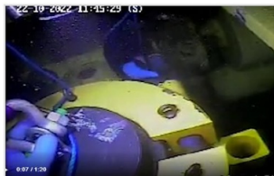
Image 2 – Diver loosening bolts
