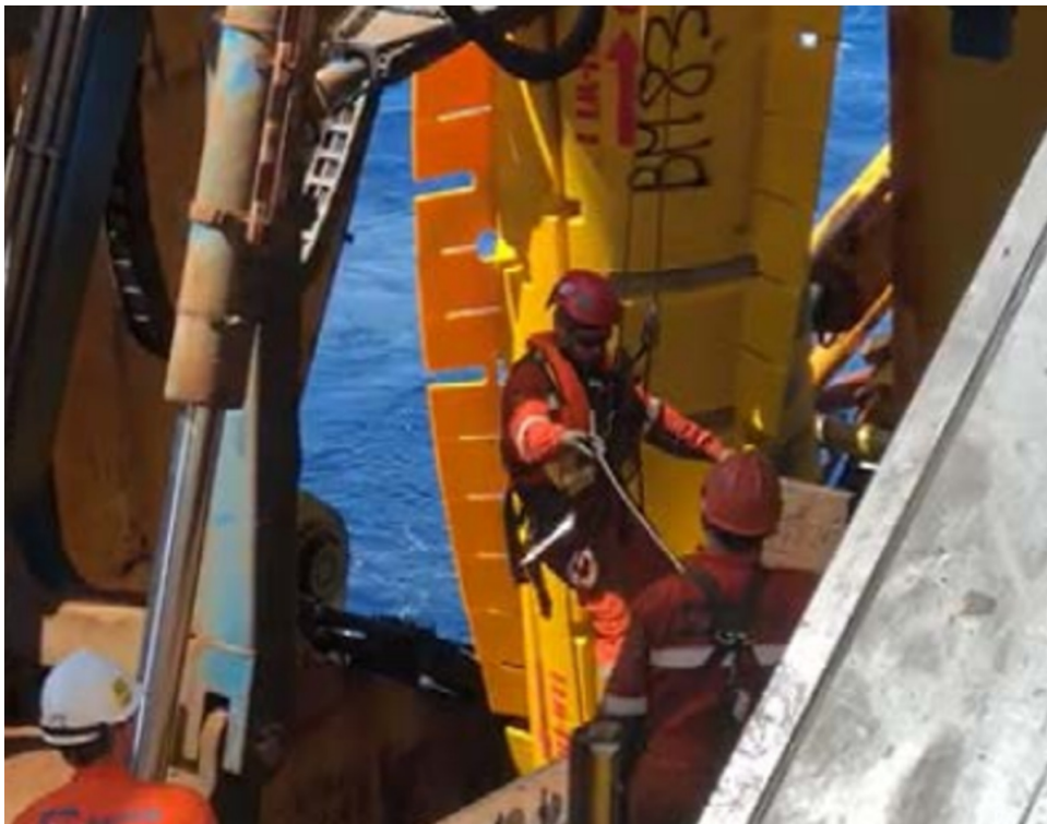
Rope access technician lost grip after stepping on slippery handrail
