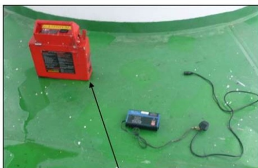
Failed unit and charging cable
