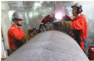
Image 1: Showing position of Technicians when handling scanner belt (note: full-length gloves shown in image not worn at time of incident)
