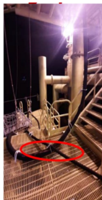
Position of temporary hoses at incident scene
