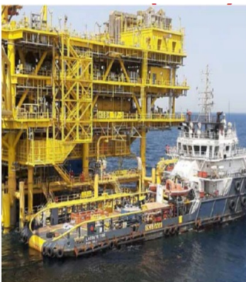
Offshore platform where incident occurred, with workboat alongside (moored to boat-landing)
